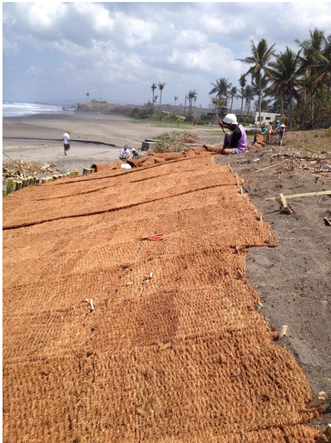
Coconut fiber geotextiles as beach revetment
